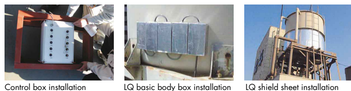
Control box installation
