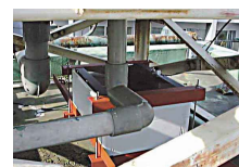
Control box installation
